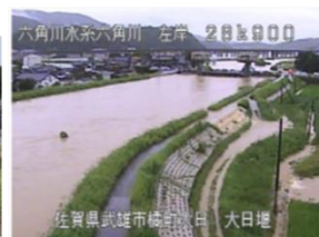
Overflow and Inflow (Rokkakugawa River)
